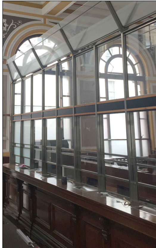
⑥ GLAZED SCREEN CAREFULLY REMOVED FROM COUNTER TOP
